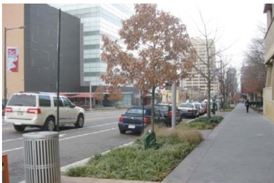
Tree trenches can accommodate multiple trees and may be connected to an underground infiltration structure.
