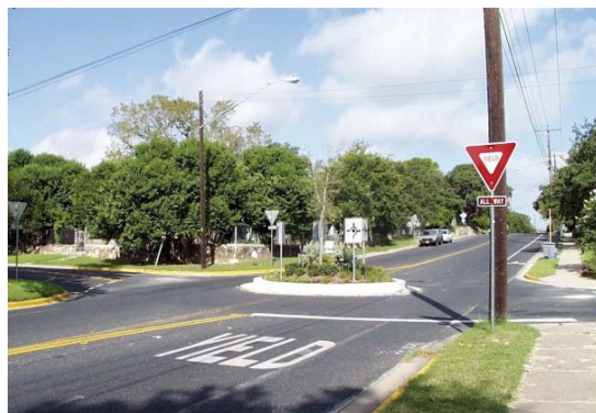
Several cities have had dramatic reductions in pedestrian crashes on local streets by installing neighborhood traffic circles (Austin.metblogs.com)
