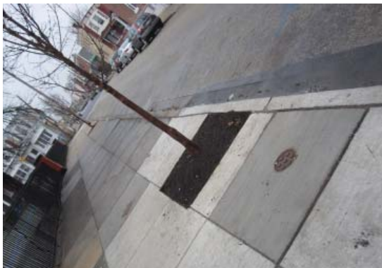
Tree pits should maintain adequate clear walking space and provide room for trees to grow without pushing up adjacent pavement such as this tree pit at the Hannity School at 56th and Webster.
