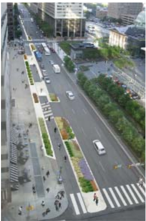
The above rendering of a proposed Center City Philadelphia Cycle track (Image courtesy of Center City District ) shows how cycle tracks may be separated from adjacent travel lanes using parking lanes, raised pavement, planters, or other treatments.
