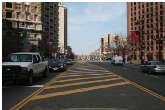
Painted medians provide some traffic calming benefits, but do not provide a protected refuge for pedestrians.
